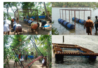
Fabrication of the "Microsate" cage by the fisherfolks
